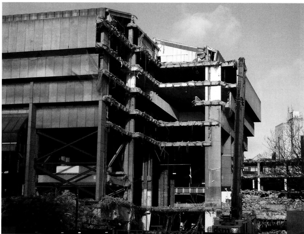
Fig.19 Demolition by 2 February 2016 Photograph by Peter Larkham
